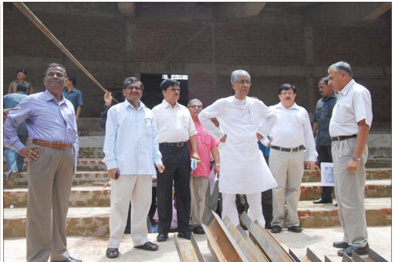
Chief Minister alongwith urban development minister and senior officials visited projects under construction in Agartala on August 18. # Pic : TO
